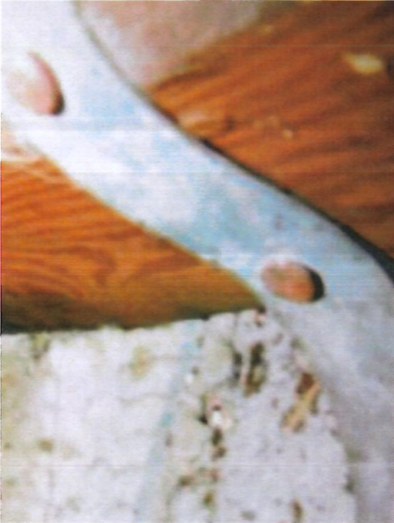
Metal Connector with 1 Nail on the Front Side & 2 Nails on the Opposing Side
