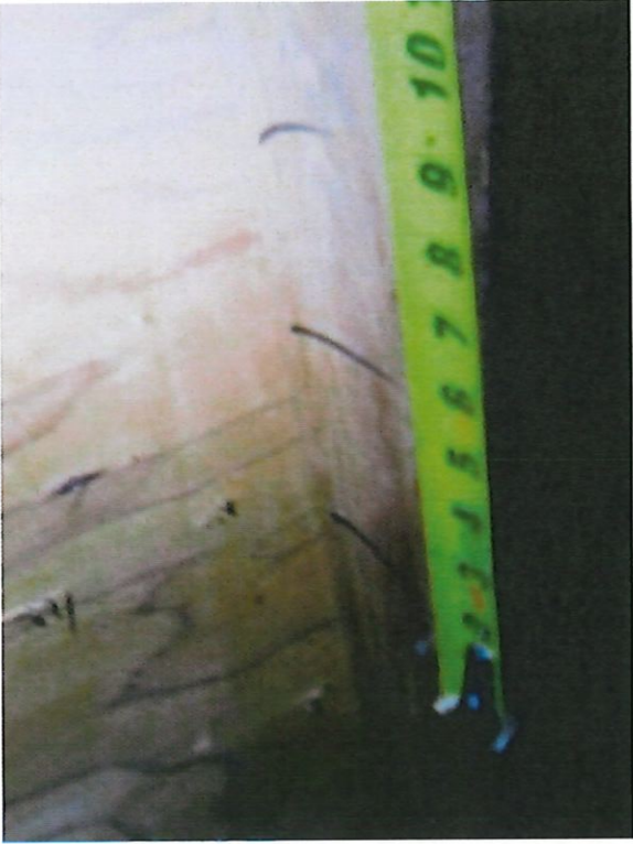
8d Nails or Greater in Size Spaced 6" in the Field
