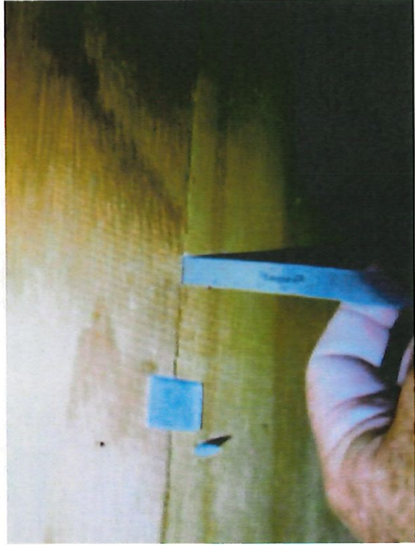
8d Nails or Greater in Size Spaced 6" Along the Edge
