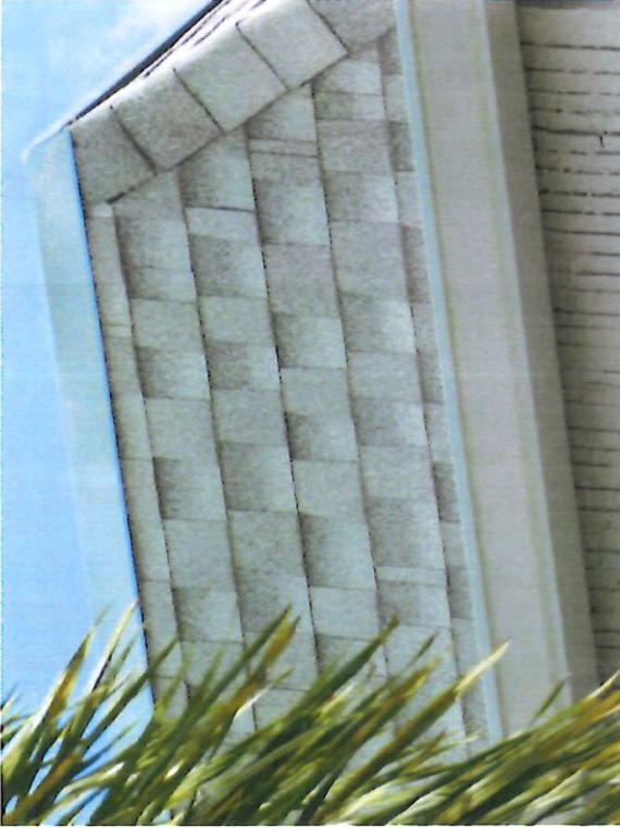
Architectural/Dimensional Shingle Roof Covering
