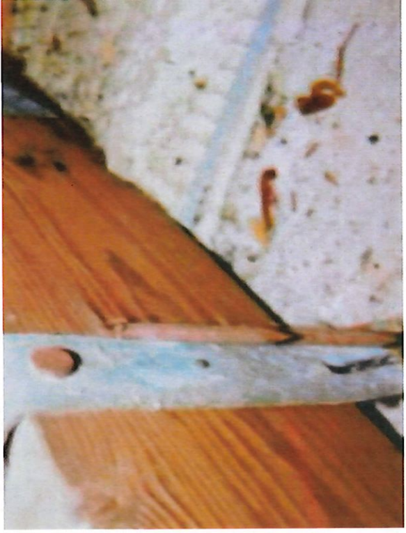
Metal Connector with 1 Nail on the Front Side & 2 Nails on the Opposing Side
